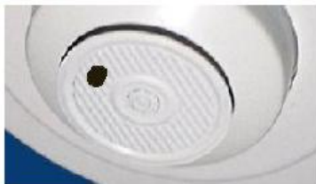
Model CF 135 W Fixed Temp. Only 135°F / 57°C Black Dot on Fin
